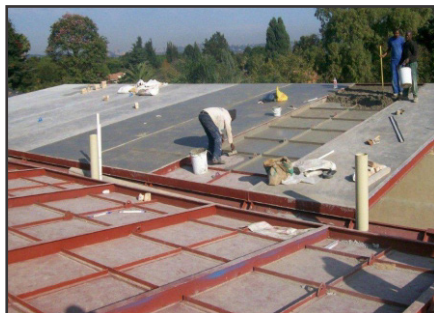
Thermally Insulating roof decks.
