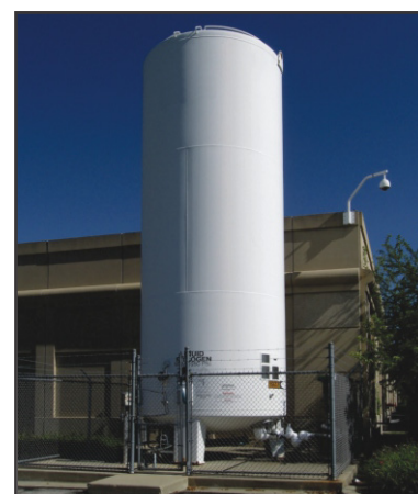
Insulating Cryogenic tanks. (Special Grade 45 Pratliperl required)
