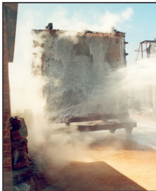
Hose stream application after one minute.
